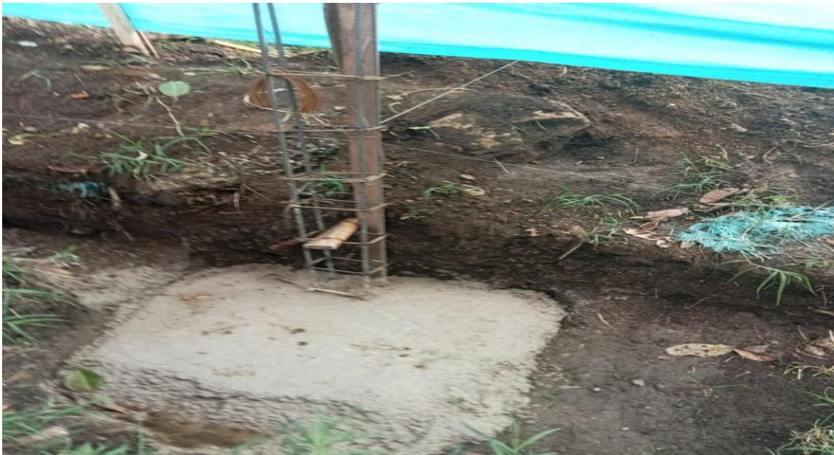
Figure 42 Zapata y columenta
