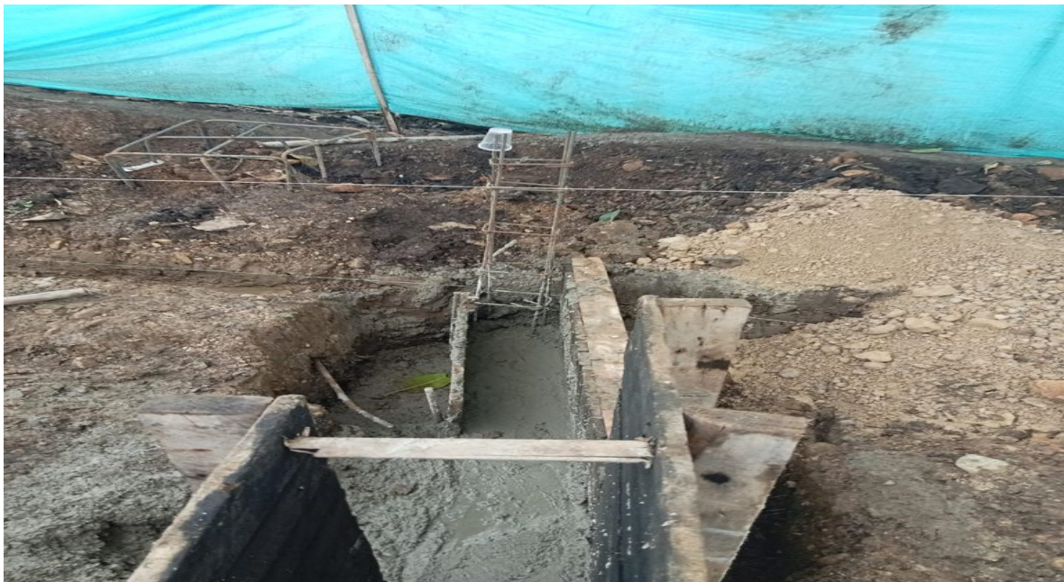
Figure 38 Fundida de zapata
