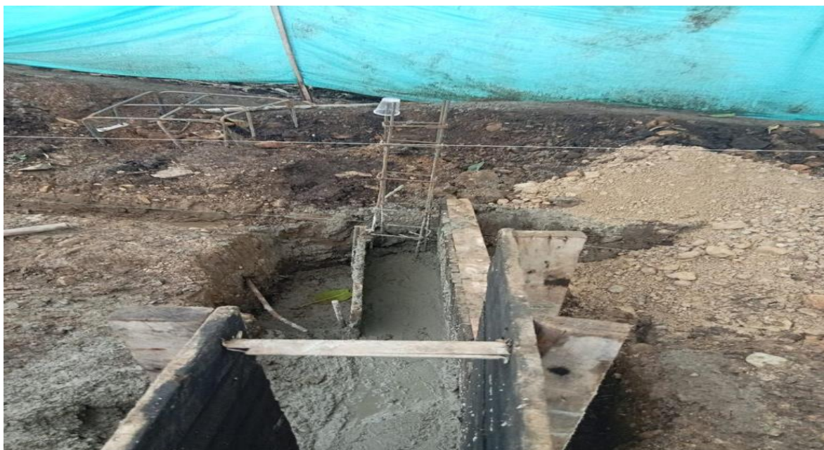
Figure 38 Fundida de zapata
