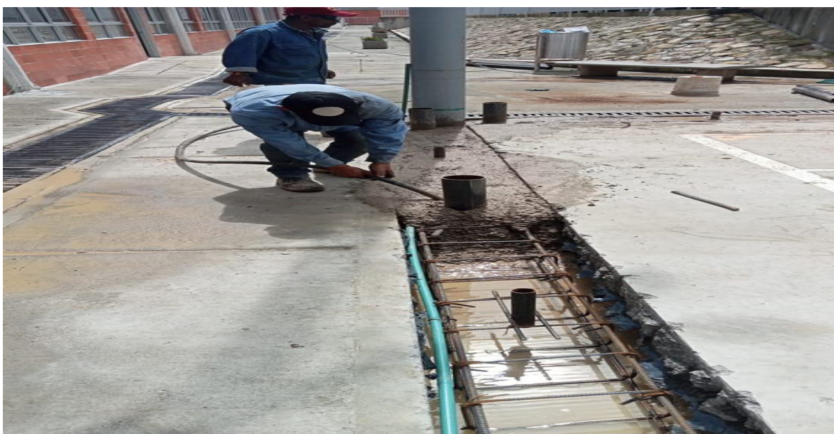
Figure 2 Fundida de concreto tremie
