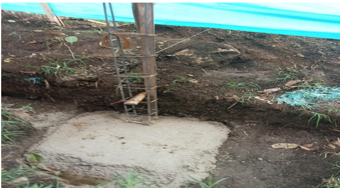
Figure 42 Zapata y columenta
