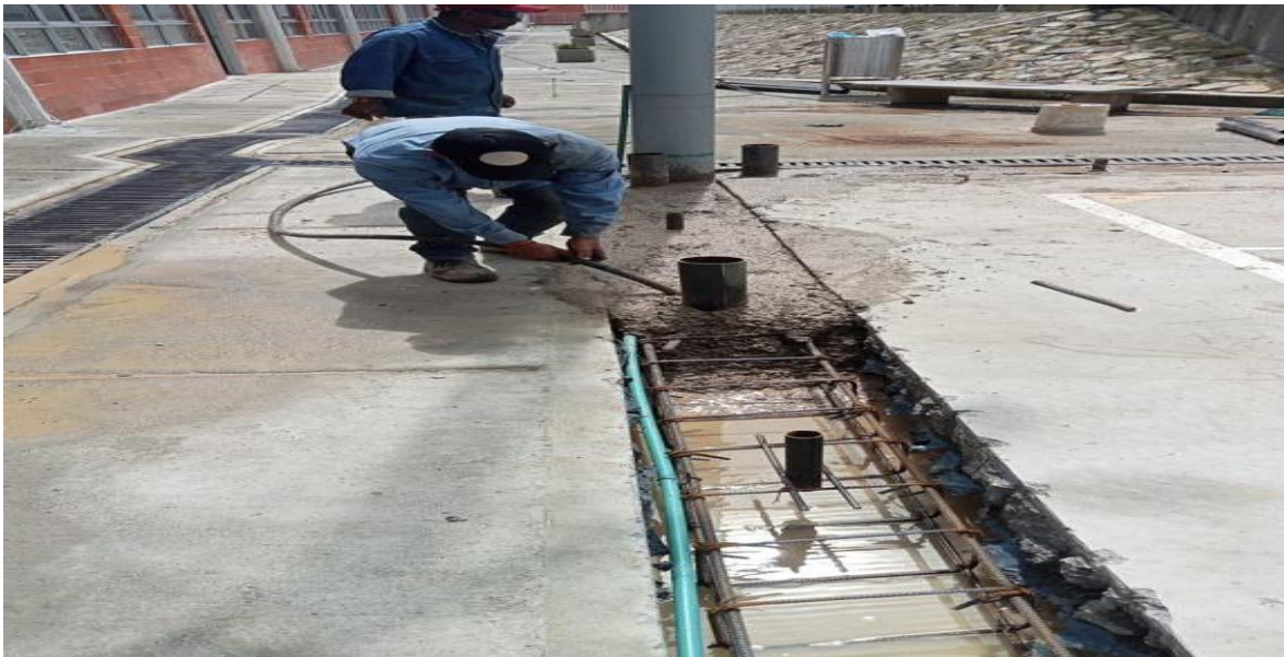
Figure 2 Fundida de concreto tremie
