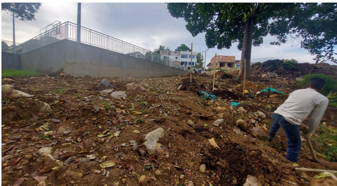
Figure 35 Replanteo y descapote
