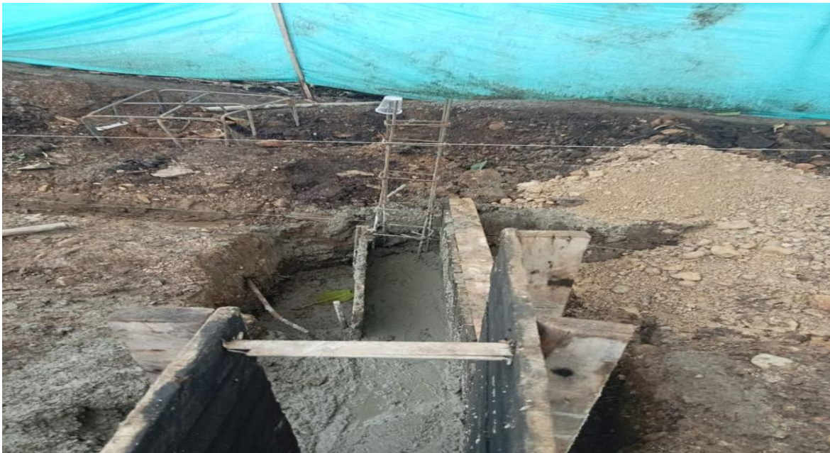
Figure 38 Fundida de zapata
