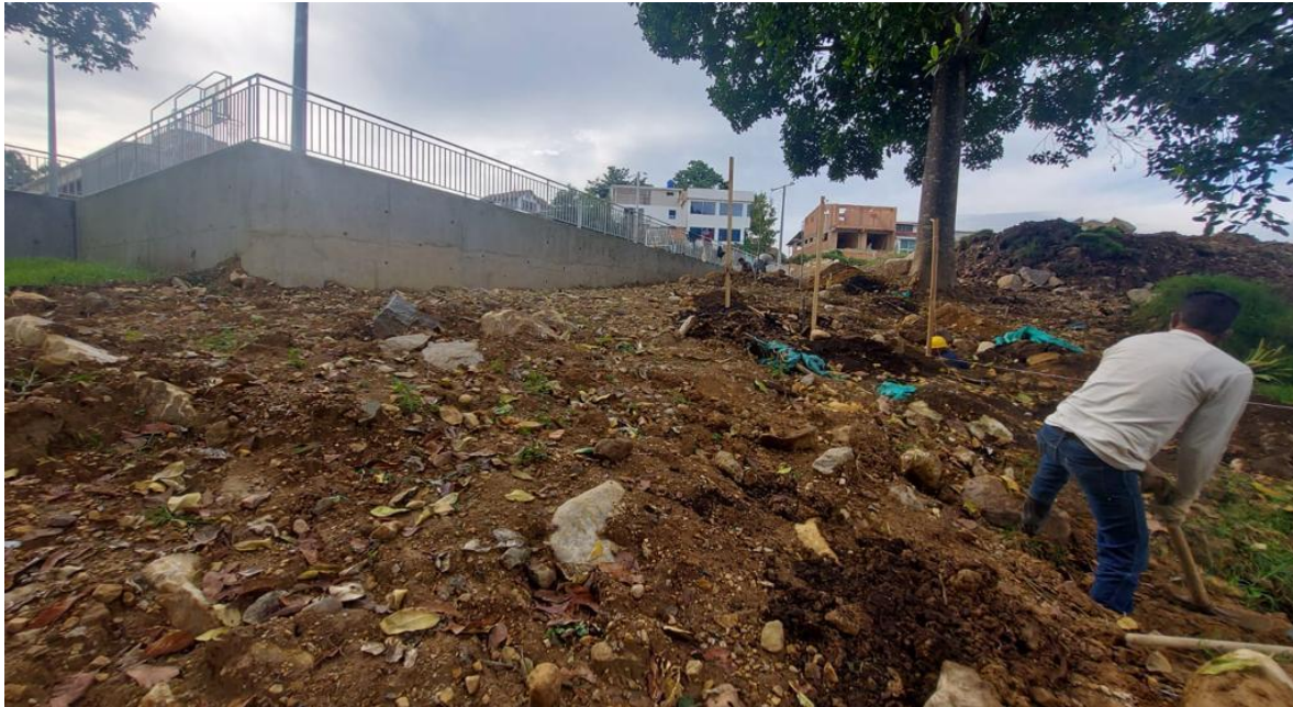
Figure 35 Replanteo y descapote
