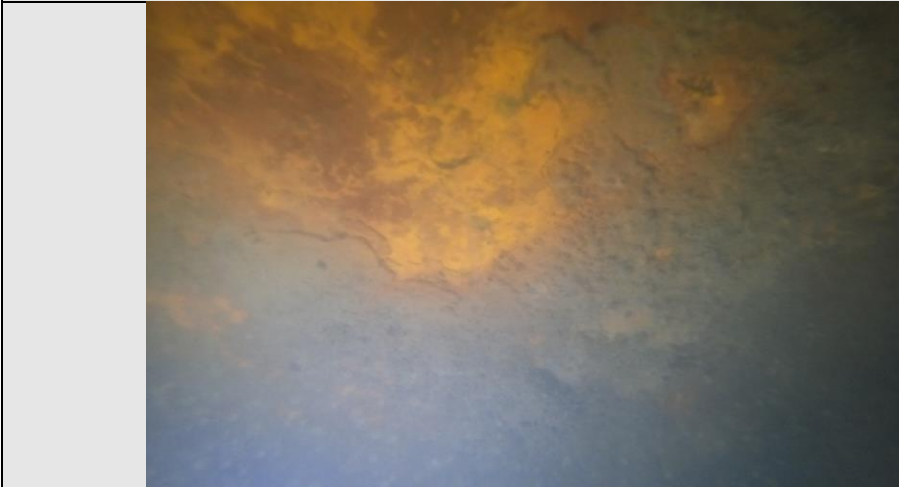
Image 4: Pile P-08 metal expose with presence of corrosion and porosity.
