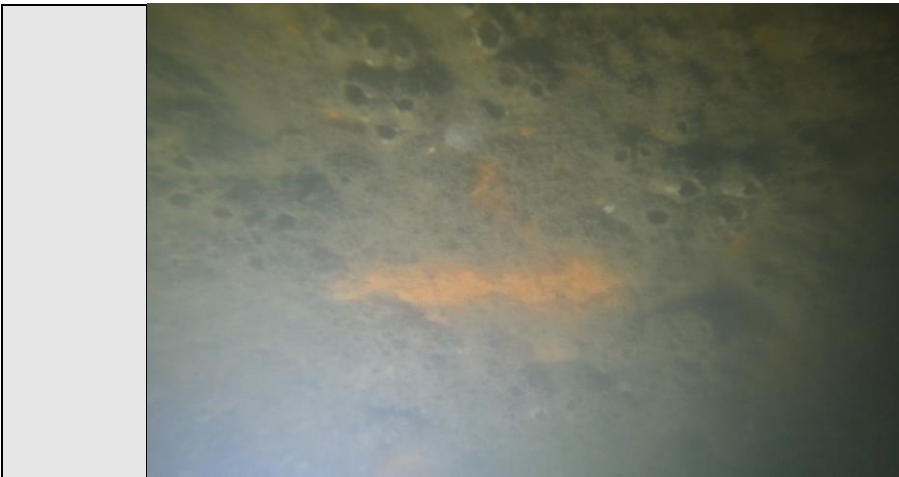
Image 3: Pile P-08 covered by marine organisms and corrosion on patches.
